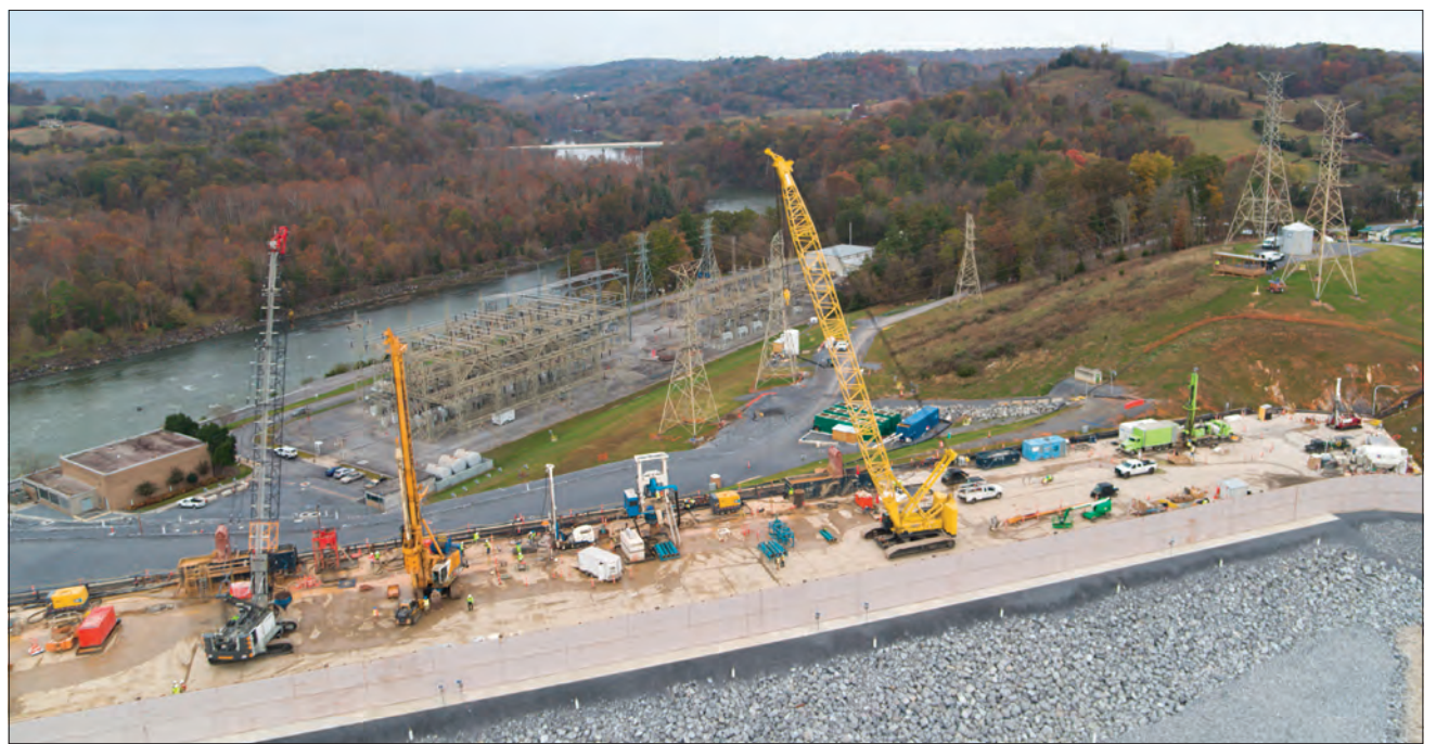
A drone shot of the construction taking place on the earthen embankment next to Boone Dam. Crews have been working to complete a cutoff wall, which was designed to provide a long-term solution to seepage problems.
