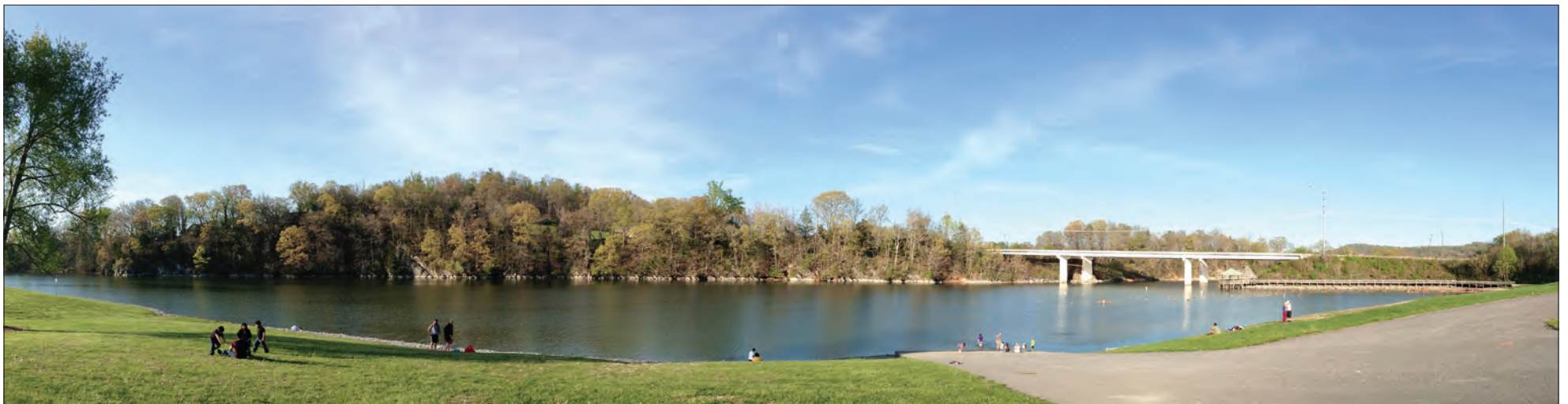
A section of Boone Lake at Winged Deer Park as it appeared in April of 2014. In October of 2014, a sinkhole was found near the base of an embankment at Boone Dam, which has forced an extended drawdown of Boone Lake in recent years. Last week, TVA officials expressed optimism that the reservoir could be filled at or near its ordinary high water mark next summer. PHOTO BY DAVE ONGIE
